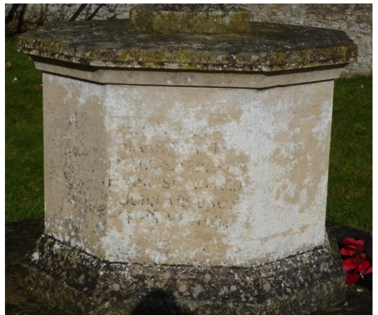
South base – names badly eroded
